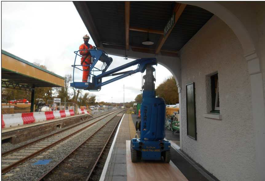
Painting from a MEWP (mobile elevated work platform).
