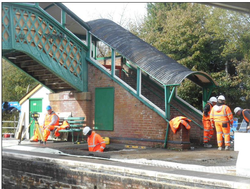
Man shows depth of light column base.
