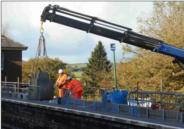
Concrete base for lighting column
