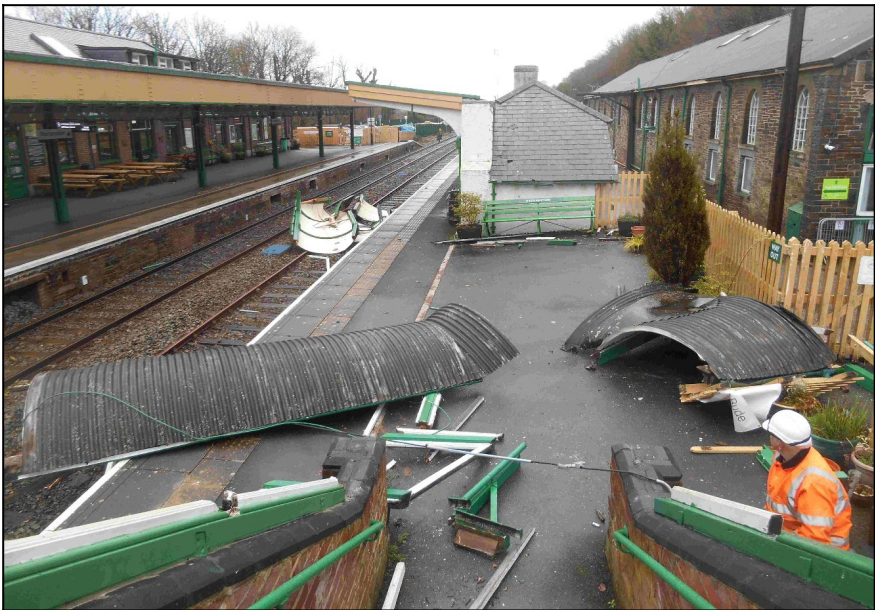
Platform 2 with debris from the footbridge
