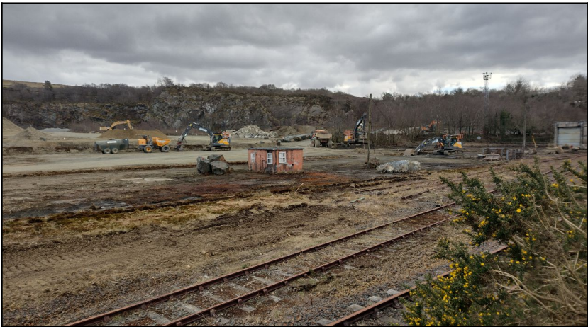
Work at Meldon Quarry on 15 th March 2025 (photo: J. Caesar)
