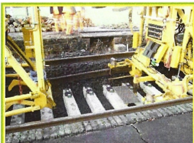
Replacement rail fed onto newly laid sleepers 17th January
