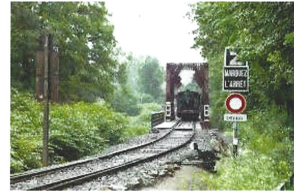
The bridge over the River Doller
