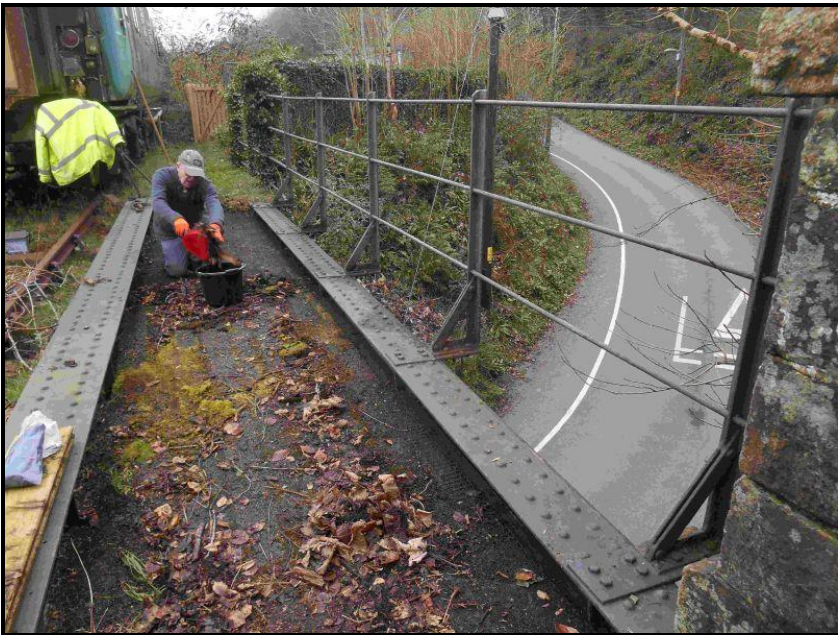
Preparing to fit the new timbers that will reduce the gap between the bridge girder and the lowest railing (Picture courtesy of Sue Baxter).
