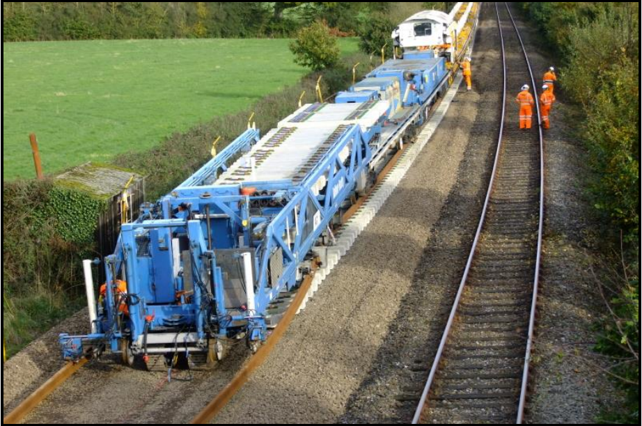
Network Rail's modern self propelled track laying machine seen at work near Yeoford on 27 th October 2019.
